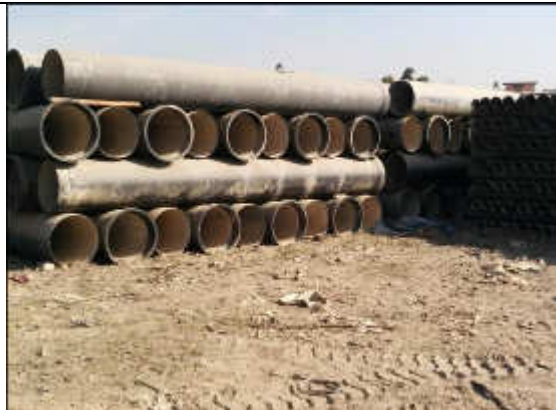
Figure 3: Pipes stockpiled at Kirtipur, Stockyard for BDS Package 1 and 2 (JITF and JWIL-SCPL)
