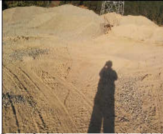
Figure 1: Sand and aggregates stocked at Arubari, BDS Package 1 (JITF)
