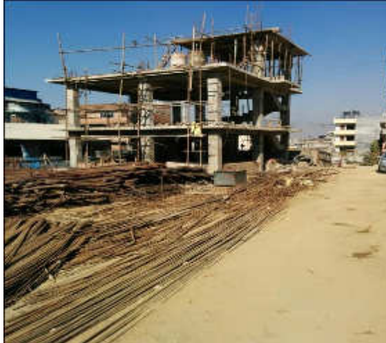
Figure 20 Work condition Khumaltar guard house, BDS Package 2
