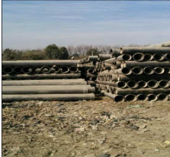
Figure 7: Pipes stockpiled at Sundarighat, Stockyard for DNI Package 3 (Sumec Lama JV)
