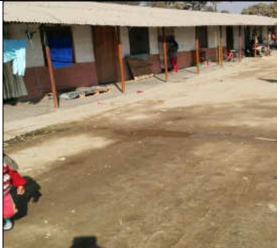
Figure 9: Accommodation building at sudarighat for DNI-3
