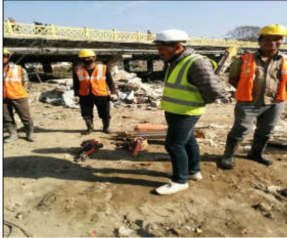
Figure 13 Work condition at site with PPEs
