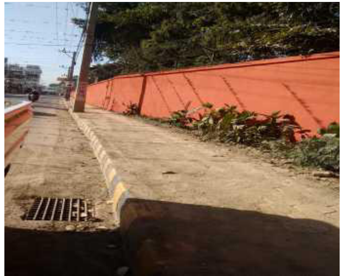
Concrete block pavement reinstatement completed at
