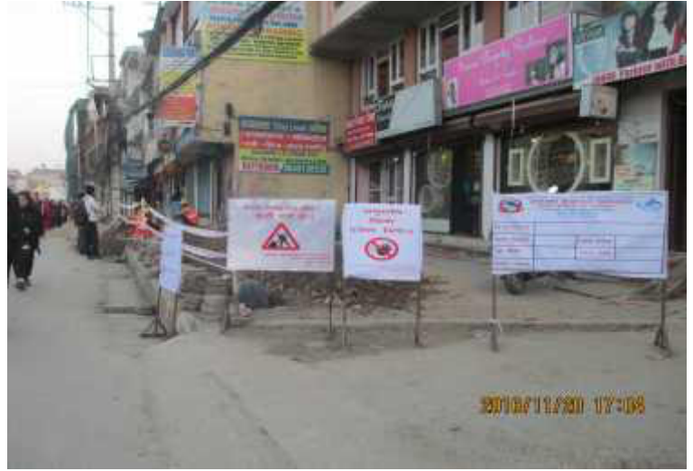
Revised Project Boards/Signage are Displayed at site
