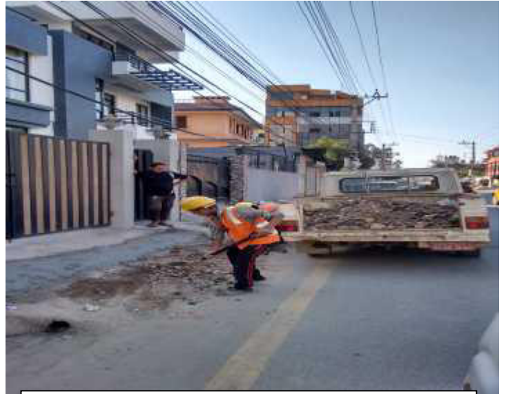
Site clearance at Sanepa,
