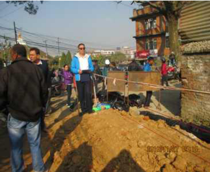
Project Director & Team leader inspected the Pipe laying site in Lalitpur
