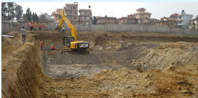
A reservoir under construction at Khumaltar in Lalitpur
