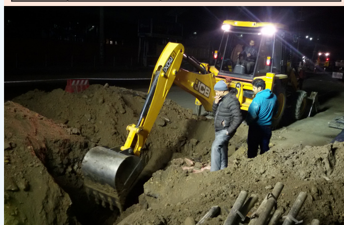
Pipes being laid from Balaju to Lainchaur during the night for the BDS
