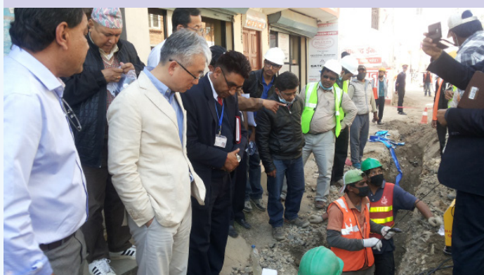
Mr Hun Kim, Director General of the ADB inspecting the pipeline laying.
