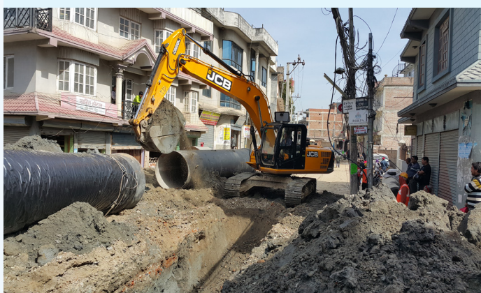
Pipeline being laid at Mahankalchaur under the BDS
