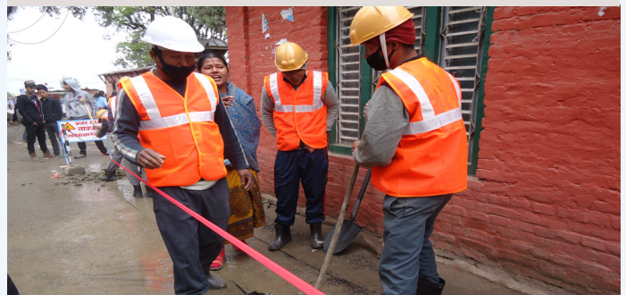
Workers using safety materials during construction work.)
