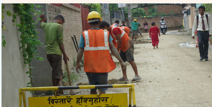
Pipeline being laid in Kathmandu as part of improving the distribution network
