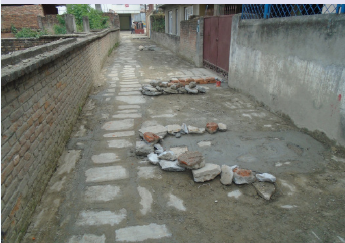
A restored lane at Anamnagar following the completion of laying pipes.
